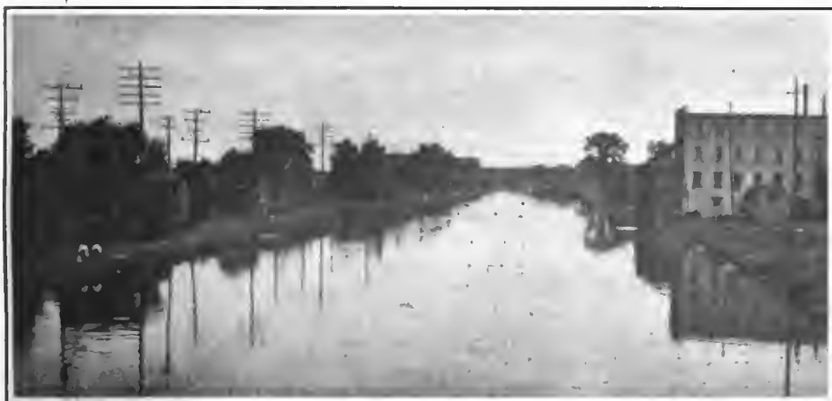
OLD ILLINOIS CANAL, NEAR LOCKPORT, ILL. NOW DISUSED
